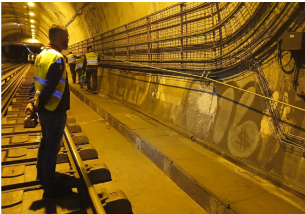
Pulling and installation of multicore fibre cable in the tunnel of the Yellow Line of the Lisbon Metro
